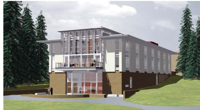
Potential Site – KIPAC building at SLAC
