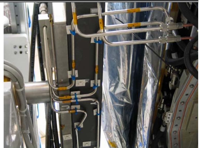
Grid chiller bar installation
