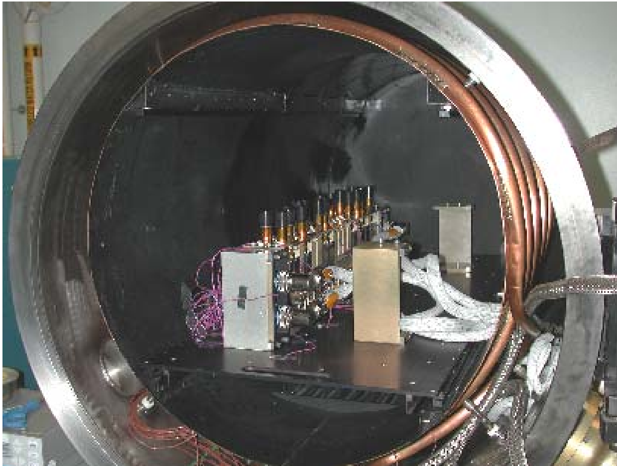
Qualification Electronics Chassis in Thermal Vacuum Chamber
