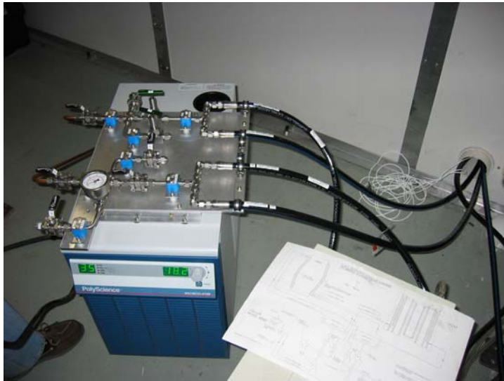
Grid Chiller Unit Installation
